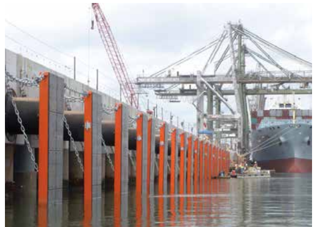
Barbour's Cut Container Terminal | Houston, TX | USA
