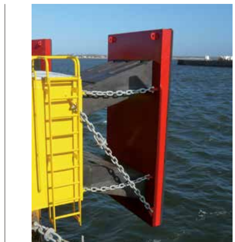
Ferry & RoRo Terminal | Rostock | Germany
