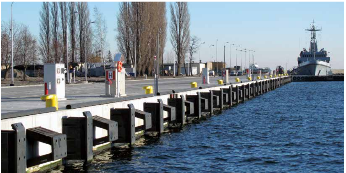
Northern Berth 16 | Port of Gdynia | Poland
