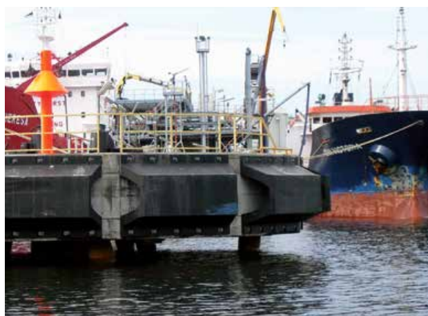
Oil Terminal | Muuga | Estonia
