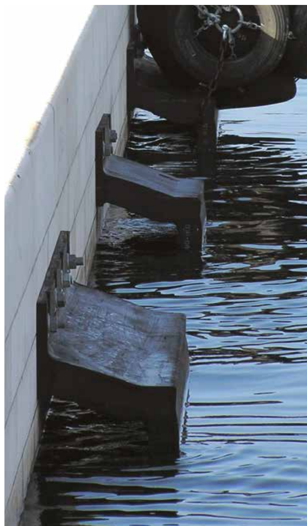
Passenger Terminal | Rijeka | Croatia
