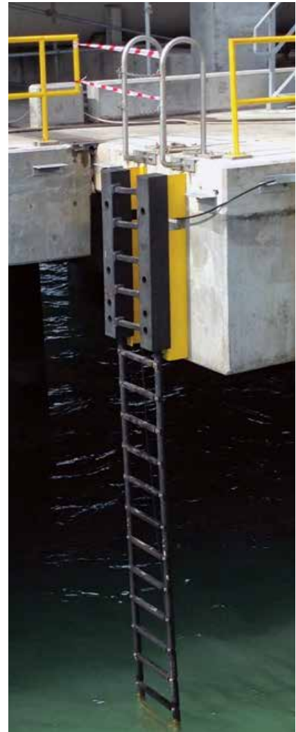
IDPT Jetty 1 | Johor | Malaysia
