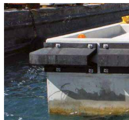
Coast Guard Terminal | Puerto Rico
