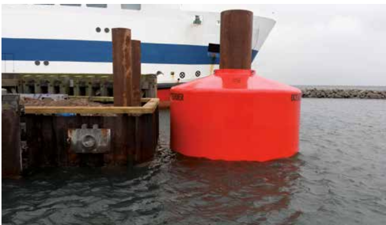
Ferry Terminal | Sejerø | Denmark
