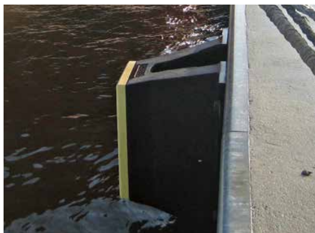
General Cargo Terminal | Amsterdam | The Netherlands
