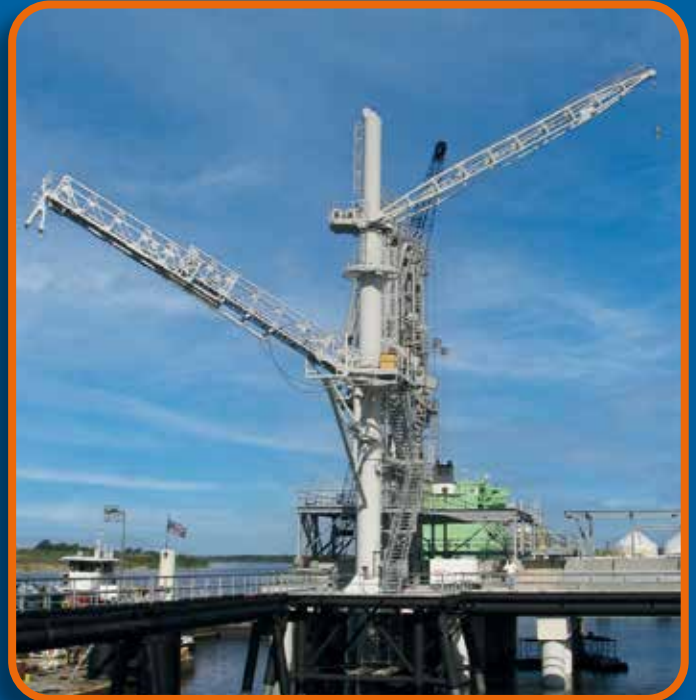
Column with telescopic access ladder and stores crane. Lake Charles - USA
