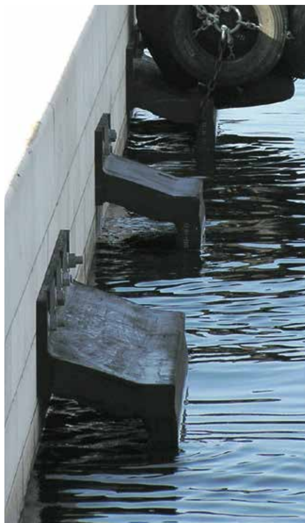
Passenger Terminal | Rijeka | Croatia
