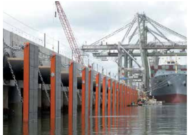
Barbour's Cut Container Terminal | Houston, TX | USA
