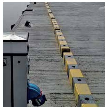
Southern Quay Wall | Simaisma | Qatar
