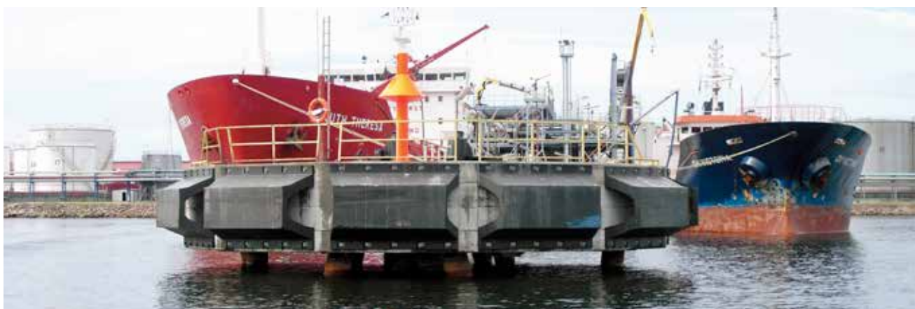
Oil Terminal | Muuga | Estonia
