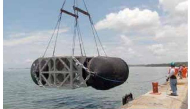
Ship Separator Installation | Guatemala
