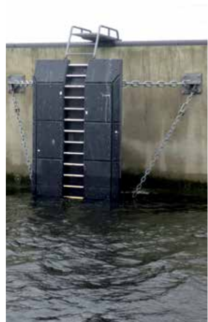
Maasvlakte II | Rotterdam | The Netherlands
