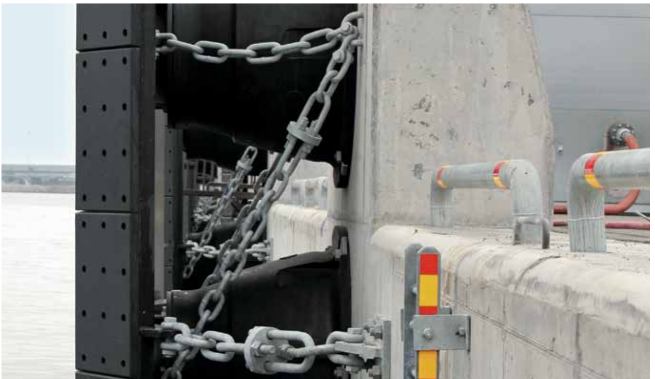
Restraint chain assemblies and brackets
