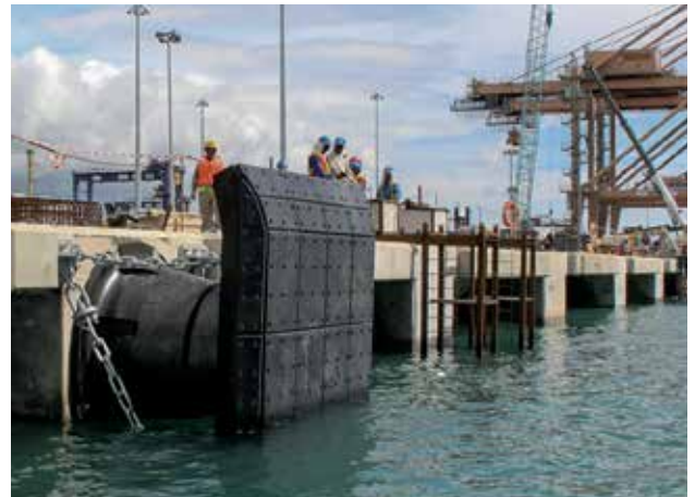
Mauritius Container Terminal | Port Louis | Mauritius
