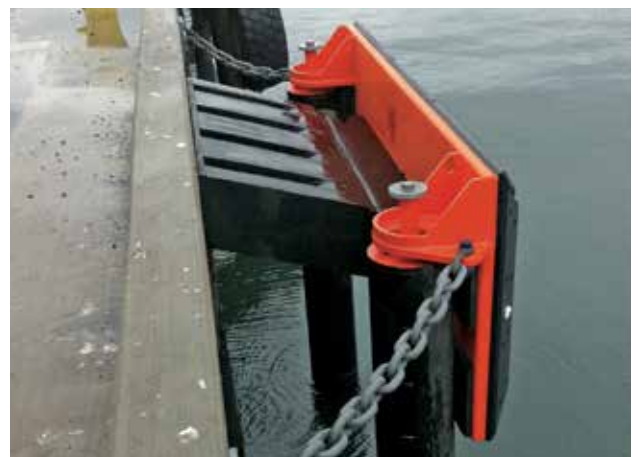
Pier 1 | North Kingstown, RI | USA
