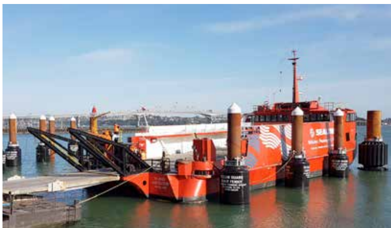
SeaLink Terminal | Auckland | New Zealand
