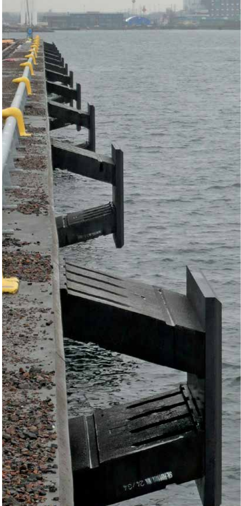
Ferry & RoRo Terminal | Malmö | Sweden
