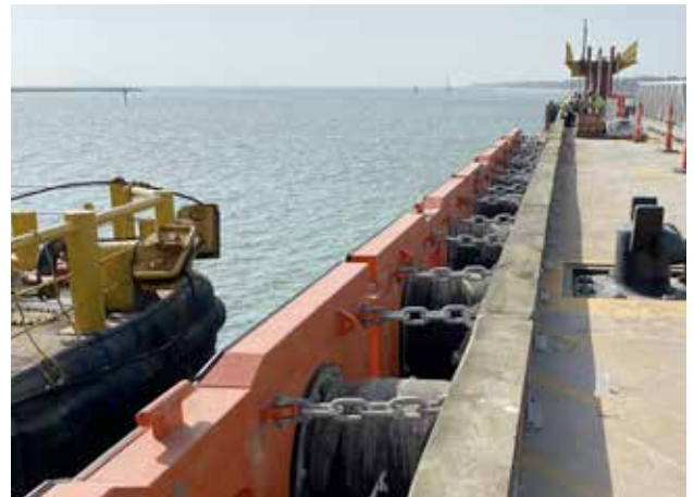
RoRo Facility | Portland, TX | USA
