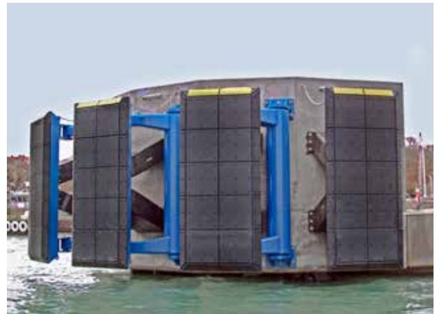
Ferry Terminal | Gotland Island | Sweden
