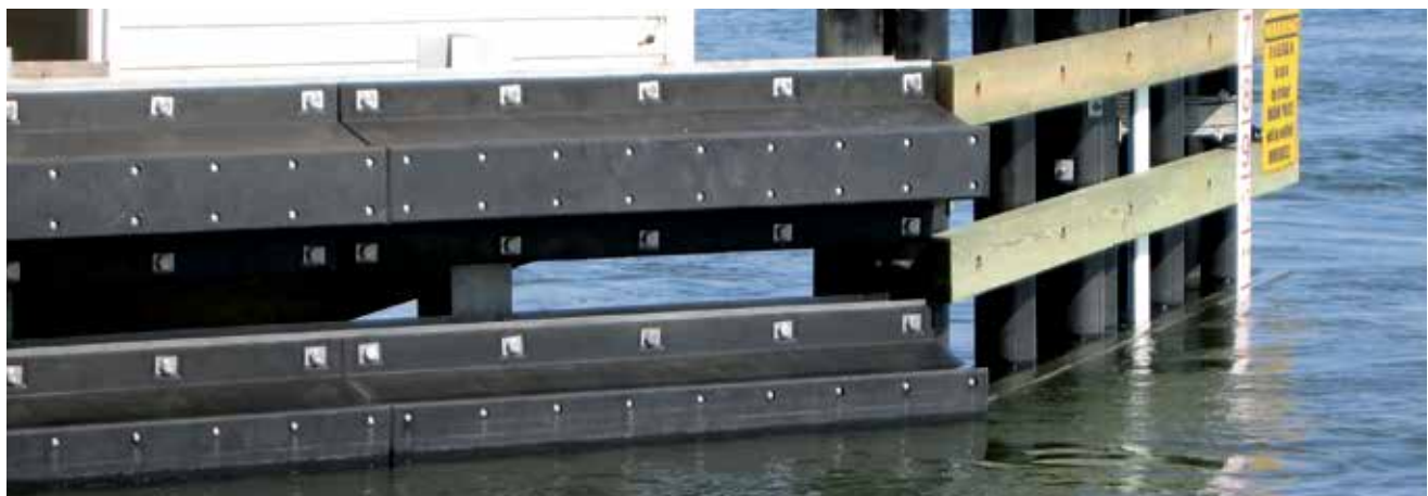
Margate Bridge | Margate City, NJ | USA
