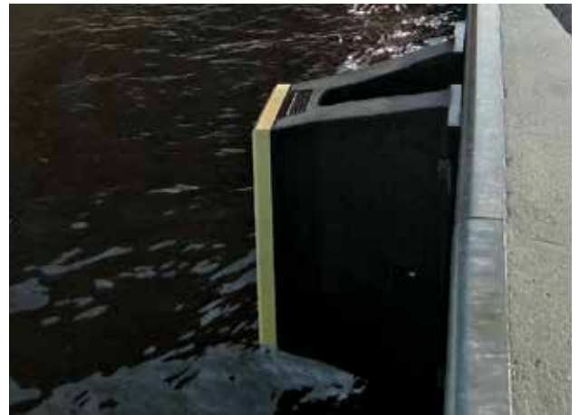
Waterland Terminal | Amsterdam | The Netherlands
