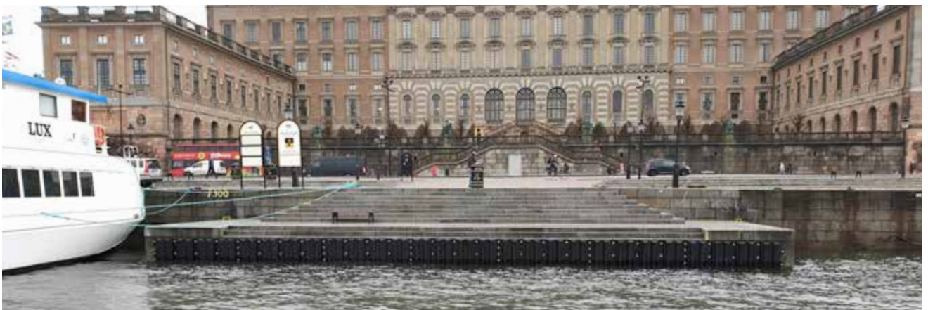
Logårdstrappan | Stockholm | Sweden
