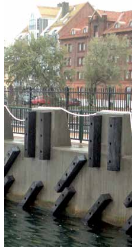
Ferry Terminal | Landskrona | Sweden
