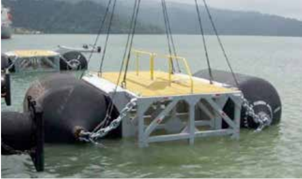
Ship Separator Installation | Guatemala
