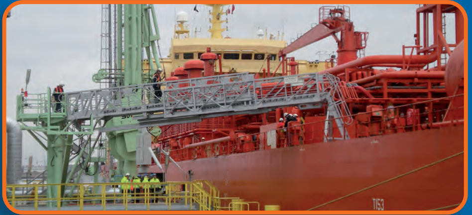
Column with telescopic gangway. Zwijndrecht - Belgium.
