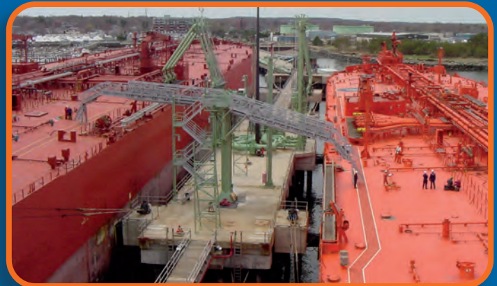
One column, with double gangway system, in Portland, Maine - USA.
