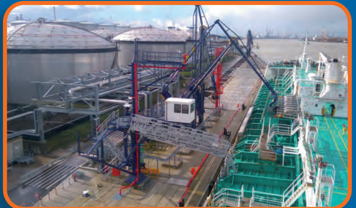
Column with telescopic ladder and cabin. Rotterdam – The Netherlands
