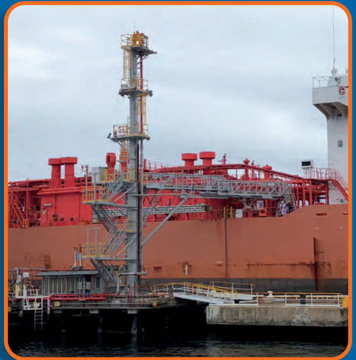
Column with telescopic gangway and fire monitor on top. Sydney - Australia.
