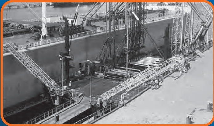
First columns with telescopic gangways, supplied in 1968. Europoort – The Netherlands.
